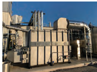
Filter Separator / Condensate Collector
