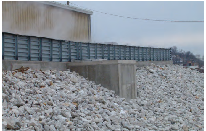
Animal Feed Supplement Odor Control Biofilter
