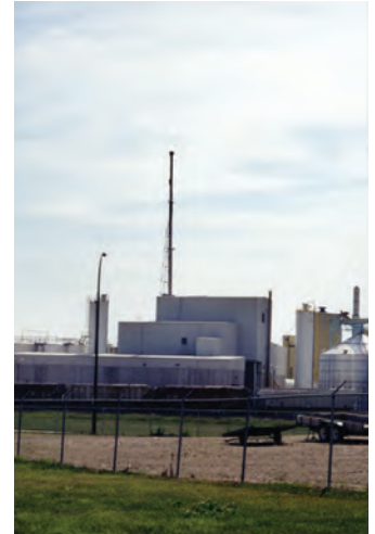
Canola Plant Facility Wide Odor Control
